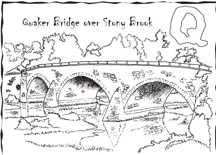
The Quaker Bridge was built around 1809 with rubble-coursed stone in an arch-barrel design. Ice breakers on the foot of the abutments collapsed in 1973, and were rebuilt along with the parapets, the low wall that protects the edge of the bridge surface where traffic travels. Also a slab was added to support heavy loads. It is one of two local bridges that played a critical role in the Revolutionary War's Ten Crucial Days Battle of Princeton. The original bridges were wooden.
